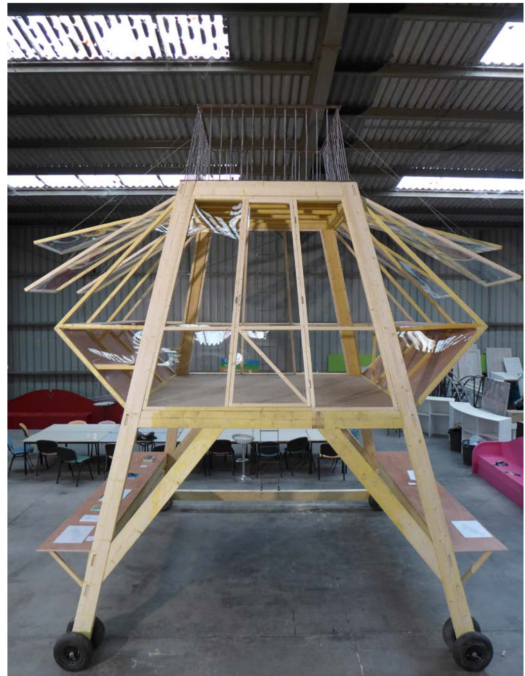
COOP 5 POUR 100 Design and construction of a mobile worksite hut. (4x4x6m) - Benjamin Le Roux - 2016
